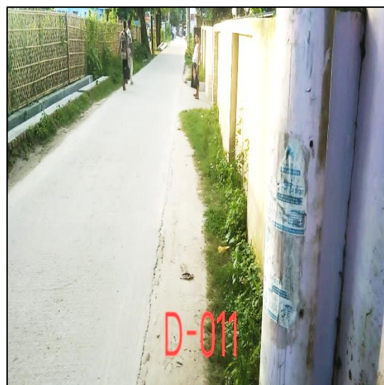
Photo , Haziganj- Drain -11
