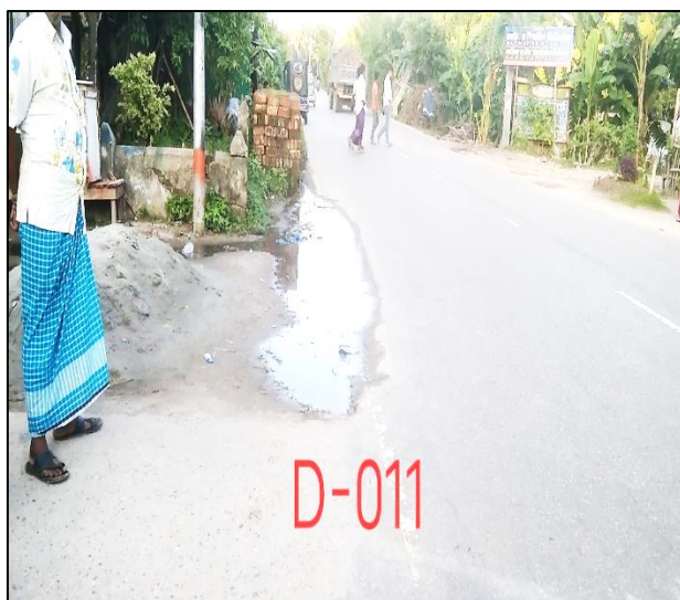
Photo , Haziganj- Drain-11
